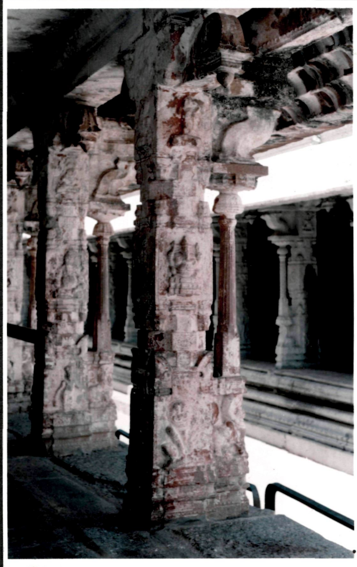
18 Columns of the south colonnade
