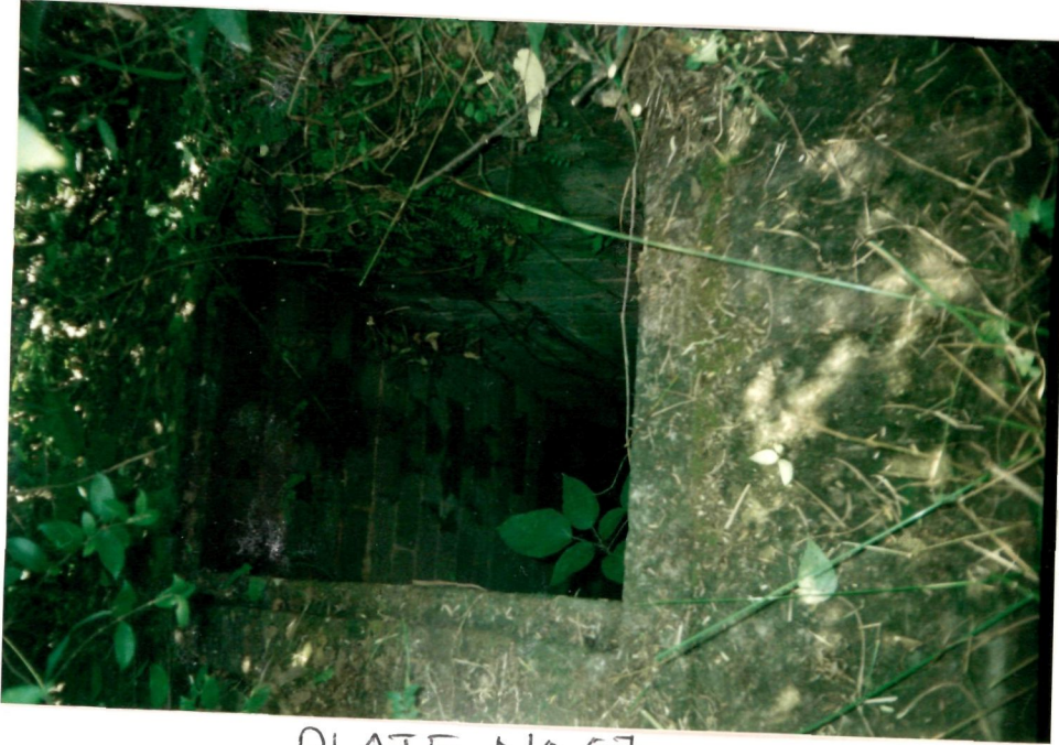
PLATE NO 57 UNDERGROUND SPILLWAY DRAIN OF WATER OF JKAPOOR SAGAR TANK.
