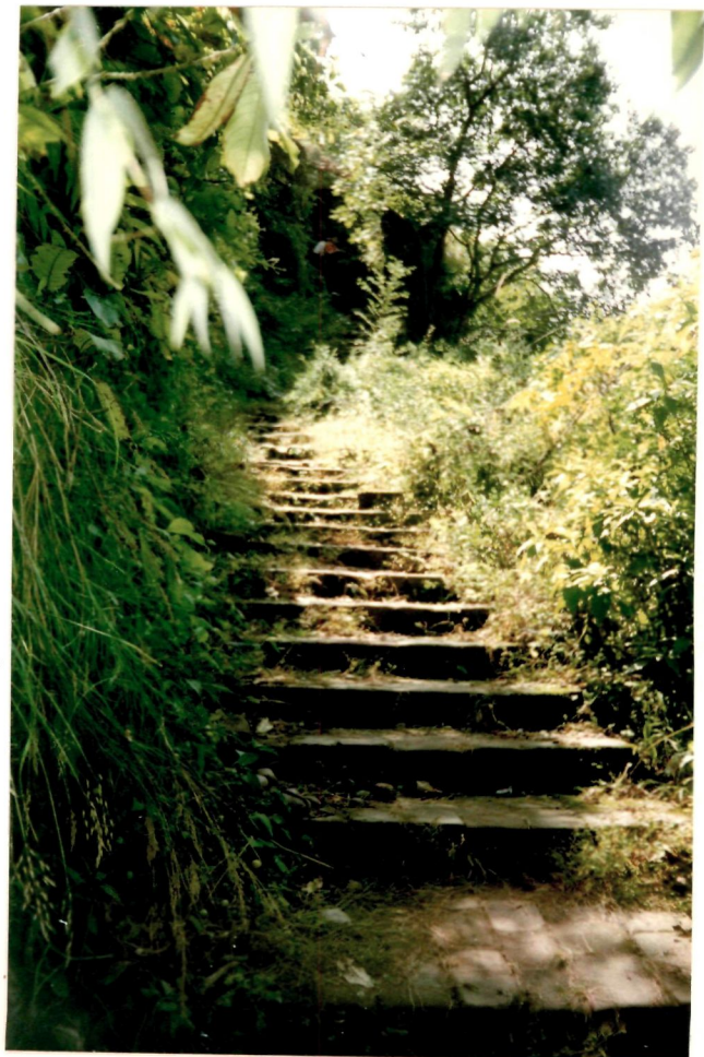
PLATE NO 52 STAIRCASE TOWARDS WESTERN DARWAZA GATE NO2 HAVING 40 STONE STEPS WITH RISE 0.25 MTRS TREAD 0.60 MTRS
