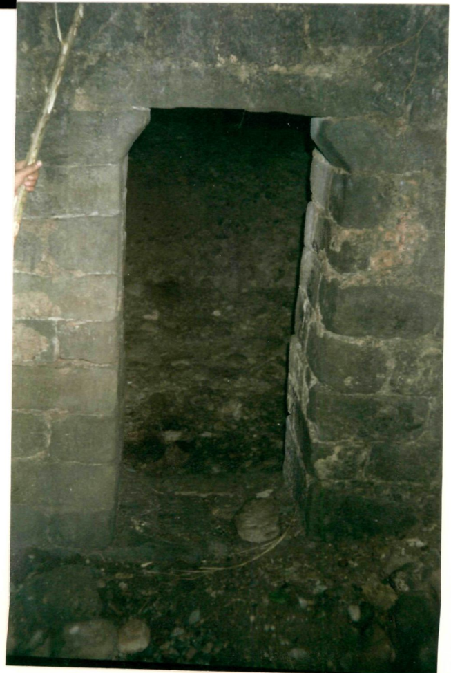
PLATE NO 48 DOOR 0.60 X 1.40 METERS OF UNDERGROUND TUNNEL OF STONE MASONRY
