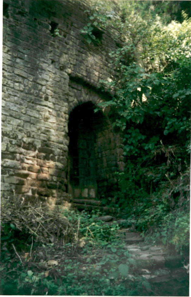
PLATE NO-55 GATEWAY OF WESTERN DARWAZA NO-I HEIGHT OF GATE IS 7.80 MTRS. DOOR SIZE 0.90 X 2.10 MTRS.
