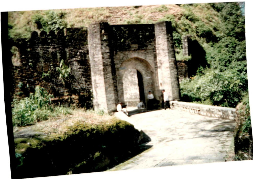
PLATE NO-6. FRONT VIEW OF RAJA RANJIT SING GATE
